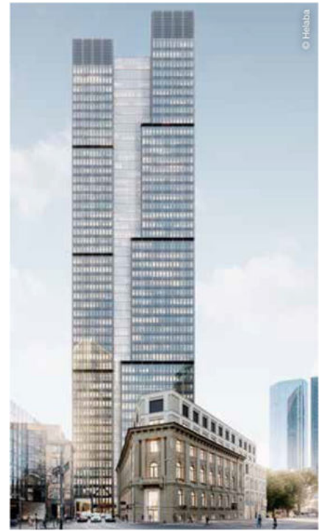
Central Business Tower
