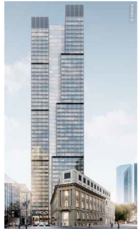
Central Business Tower
