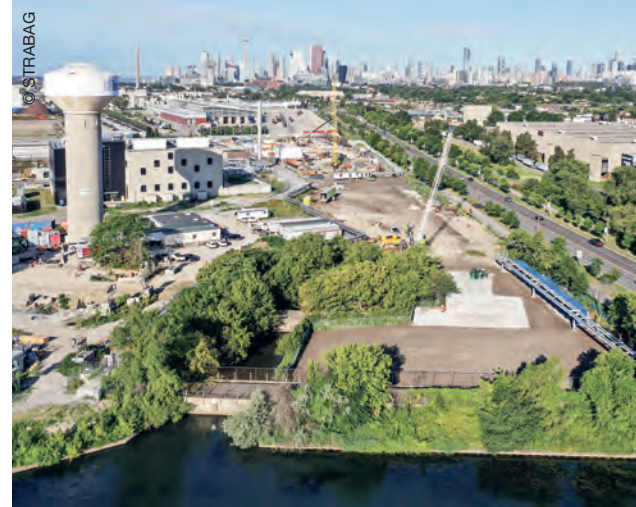
The pumping station will be built on this site of the Ashbridges Bay Wastewater Treatment Plant.
