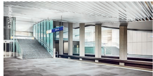
STRABAG is renovating the south section of the M3 metro line in Budapest
