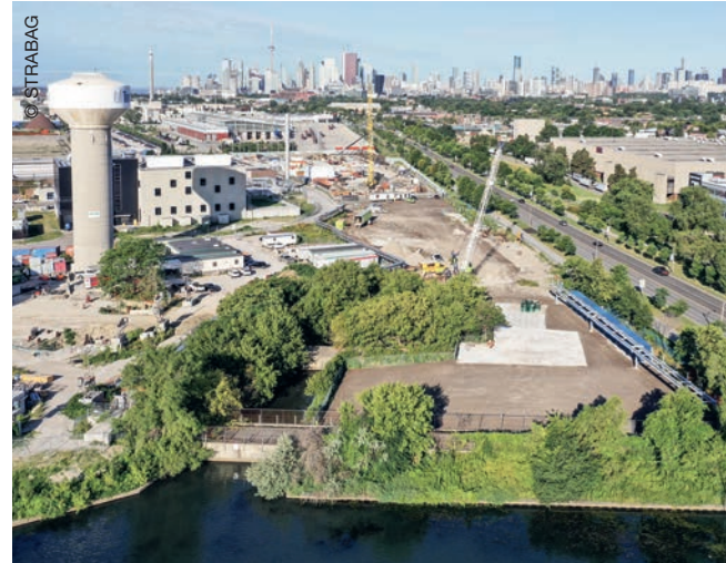
The pumping station will be built on this site of the Ashbridges Bay Wastewater Treatment Plant.
