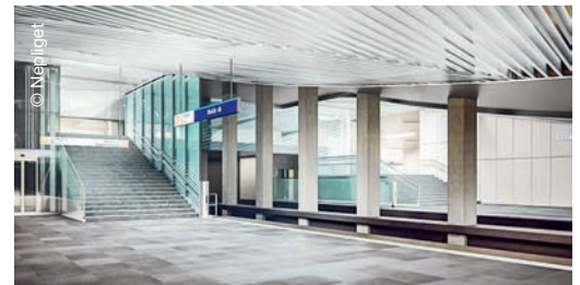
STRABAG is renovating the south section of the M3 metro line in Budapest
