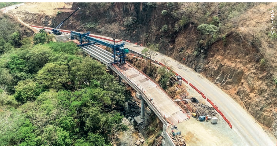
Work on the Autopista al Mar 1 in Colombia
