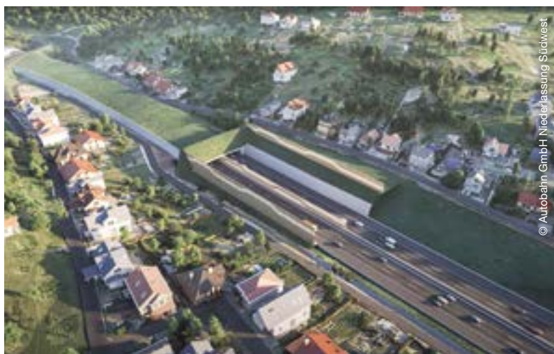
Large-scale project Enz Valley crossing
