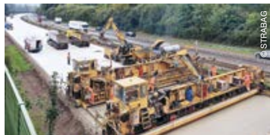
Widening of the A1 motorway
