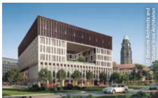
Administration centre for Dresden
