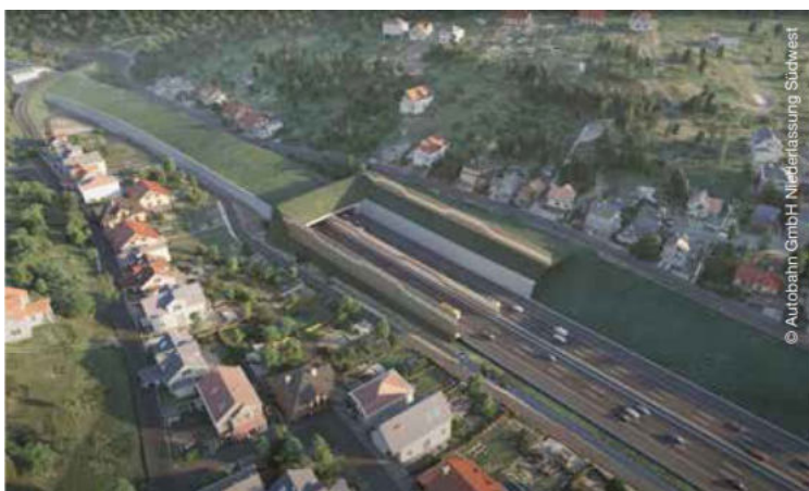
Large-scale project Enz Valley crossing
