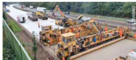
Widening of the A1 motorway.
