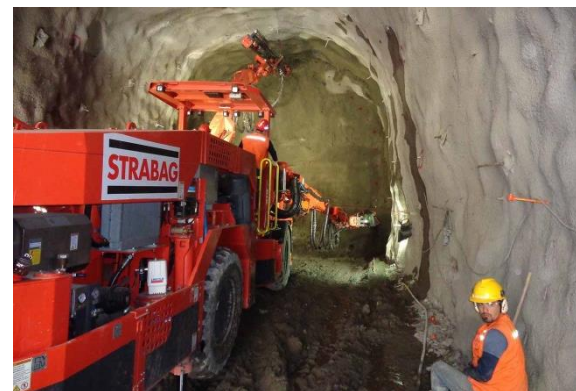
Alto Maipo power plant
