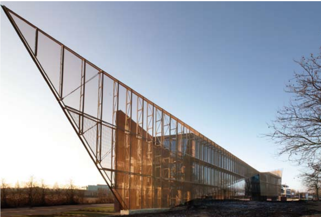
OFFICE BUILDING EIJSSEN, BELGIUM
