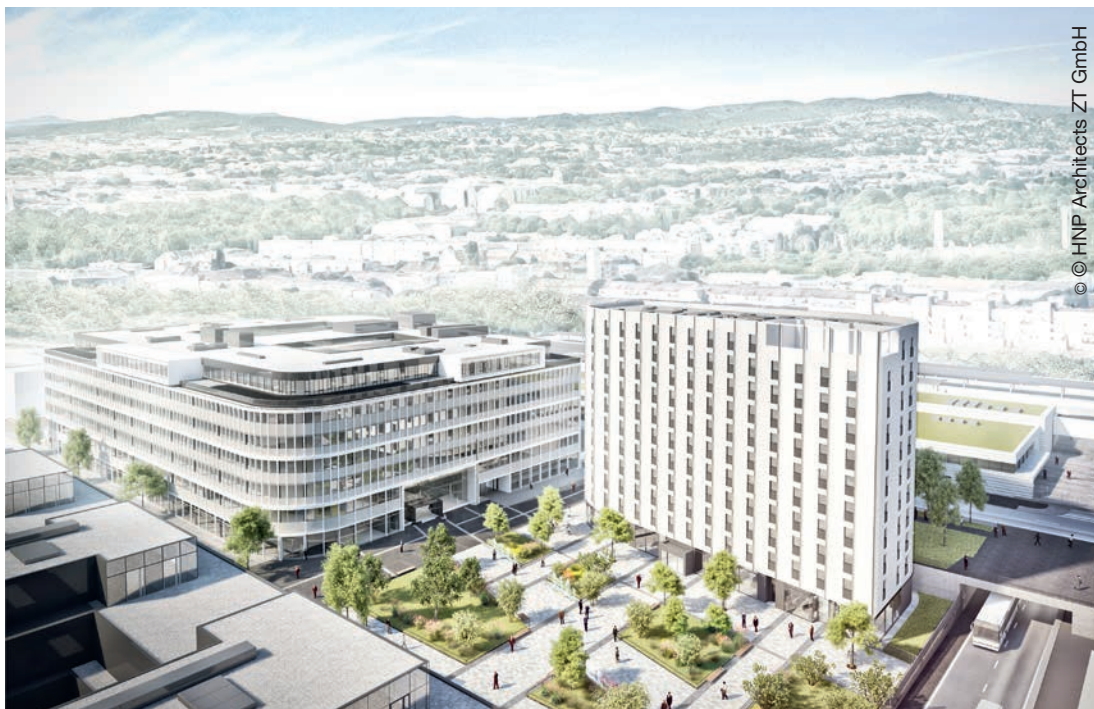
The SMARTments in Vienna, developed by STRABAG Real Estate, were awarded pre-certification in gold by the Austrian Sustainable Building Council (ÖGNI) already during the construction phase.
