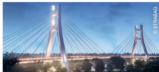
The cable-stayed bridge across the river Someș
