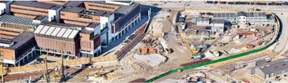
Construction of a 2 km metro tunnel
