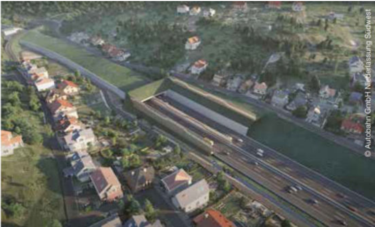
Large-scale project Enz Valley crossing
