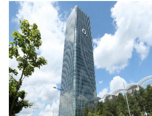
O 2 Telefonica Munich, Germany, Office, data center
