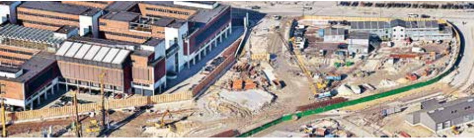
Construction of a 2 km metro tunnel
