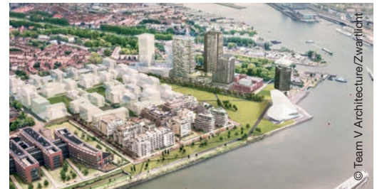
STRABAG subsidiary ZÜBLIN to build the large-scale project Congresshotel & Residential Tower Overhoeks in Amsterdam.
