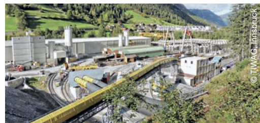
The run-of-the-river power plant on the Inn will make a significant contribution to Tyrol's energy autonomy.
