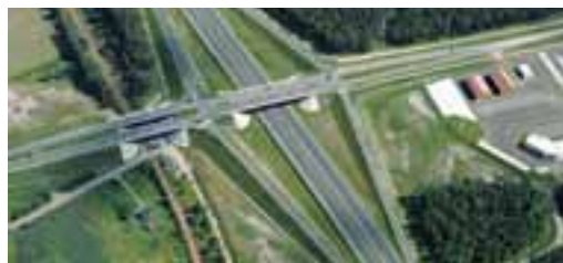
Section of A4 motorway
