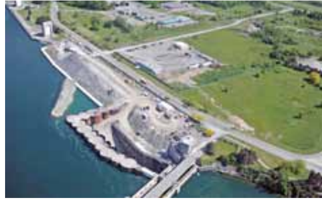
Construction of Niagara Tunnel Project
