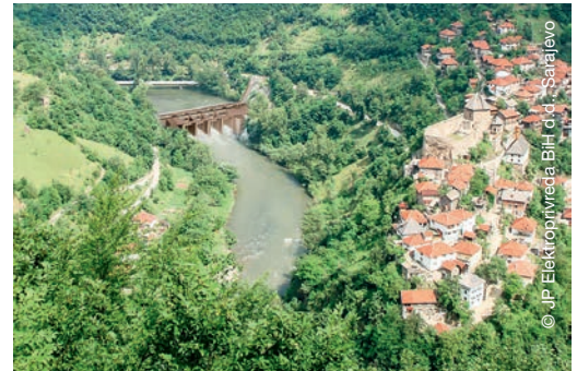
Hydroelectric power plant on the river Bosna
