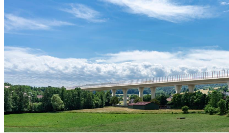
Replacement of the Utrichshausen viaduct on A7
