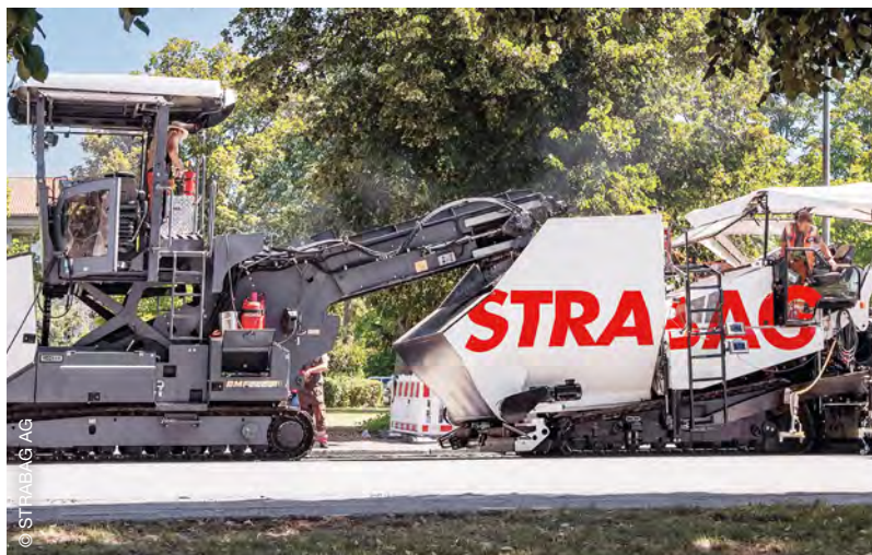
CIAir® Asphalt paving with the STRABAG AG innovation paver in Erlangen
