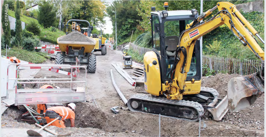
Construction work in Küsnacht (CH) with digitally accessible resident communication updated on a daily basis.
