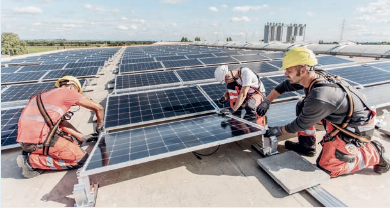
Installation of the pv system on the roof of the Mischek precasting plant
