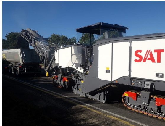
On-site recycling of asphalt
