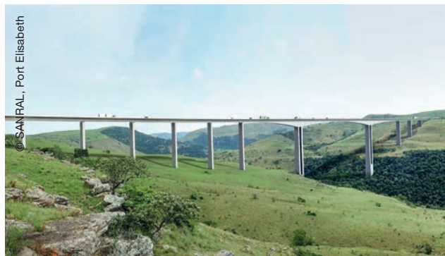
Bridge over the river Mtentu – after completion, it will be Africa's highest bridge.
