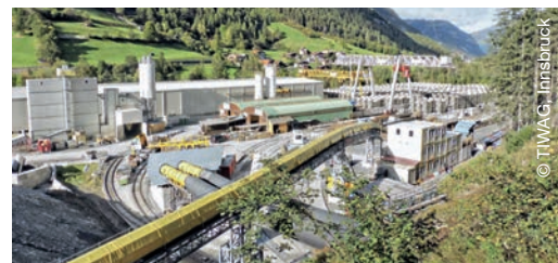
The run-of-the-river power plant on the Inn will make a significant contribution to Tyrol's energy autonomy.
