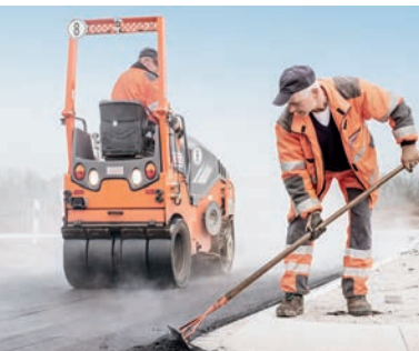
High demand in road infrastructure
