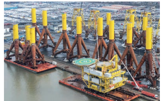
New port construction contract in Bremerhaven
