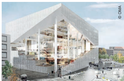
Construction under teamconcept partnering scheme
