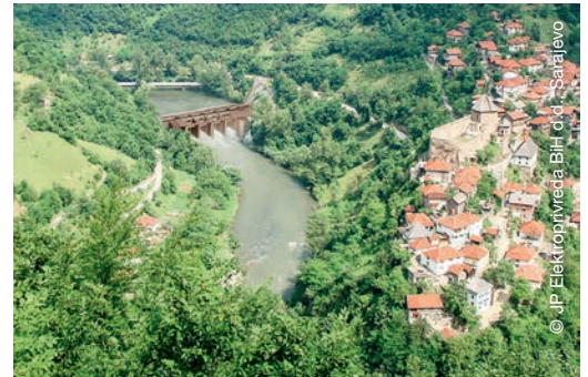
Hydroelectric power plant on the river Bosna
