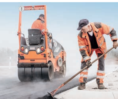
High demand in road infrastructure
