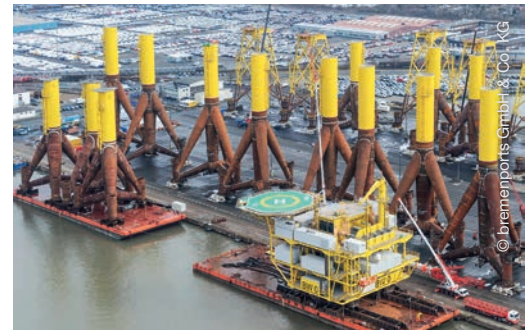
New port construction contract in Bremerhaven
