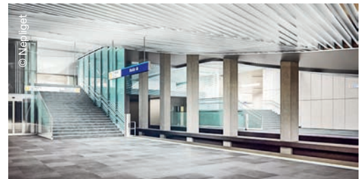
STRABAG is renovating the south section of the M3 metro line in Budapest
