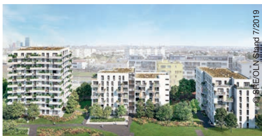
Privately financed owner-occupied flats at In der Wiesen Ost
