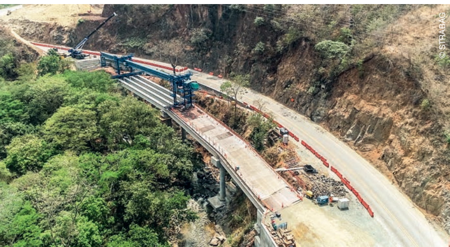
Work on the Autopista al Mar 1 in Colombia
