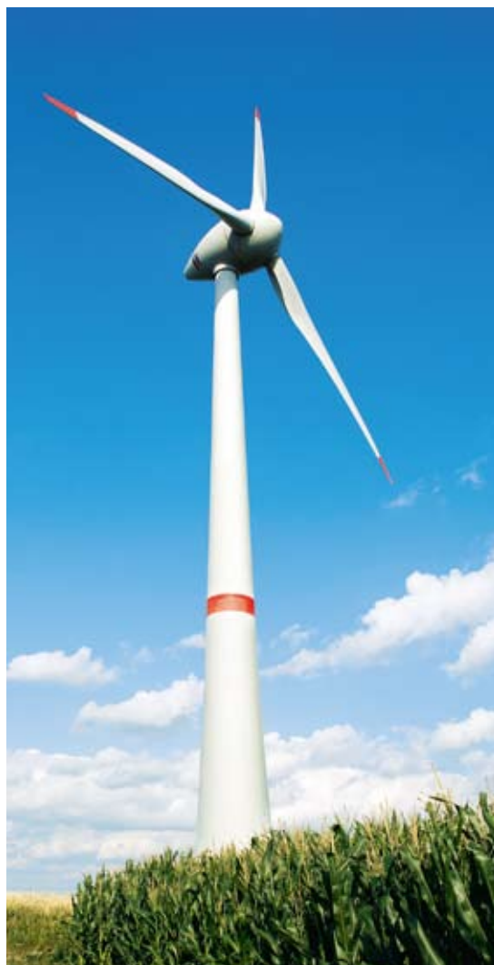
LARRELTER POLDER WIND FARM IN EMDEN, GERMANY
