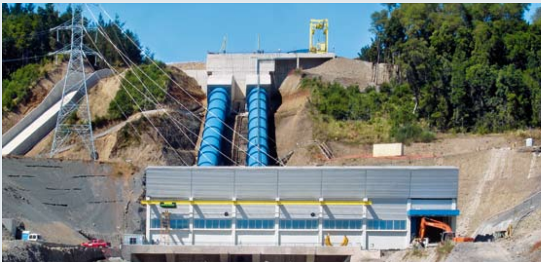
PRODUCES UP TO 464 GWH OF ELECTRICITY A YEAR
