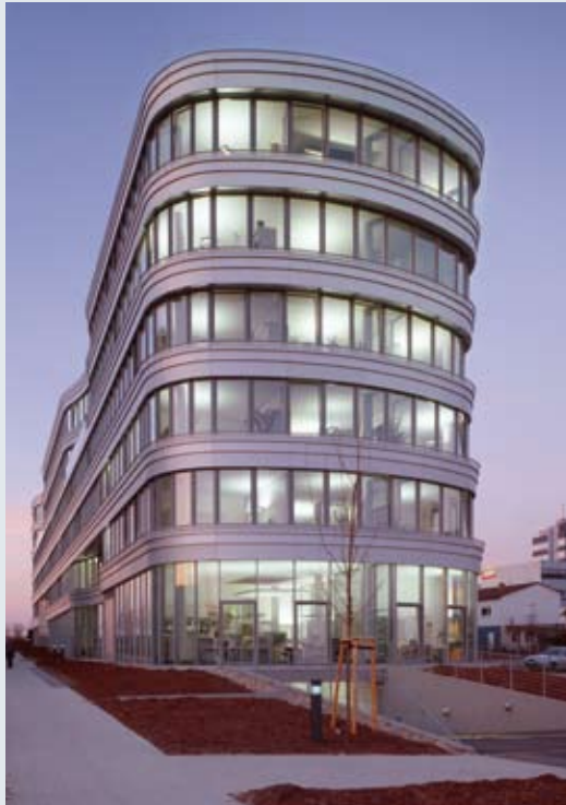
VIEW OF SOUTH-WEST FACE OF THE Z-ZWO OFFICE BUILDING
