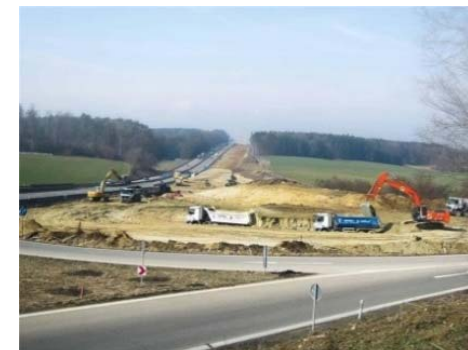
Motorway A8, Germany
