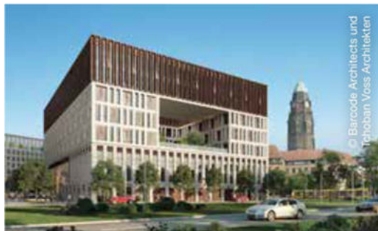
Administration centre for Dresden.
