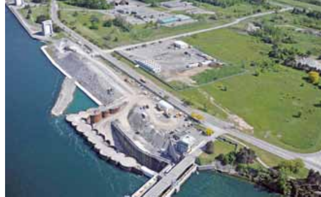
Construction of Niagara Tunnel Project
