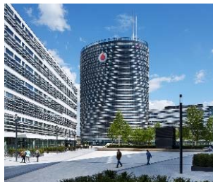
Vodafone Campus Düsseldorf, Germany
