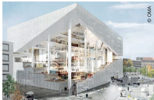
Construction under teamconcept partnering scheme
