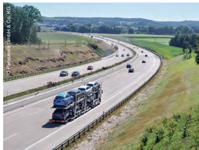
View of the A8 motorway
