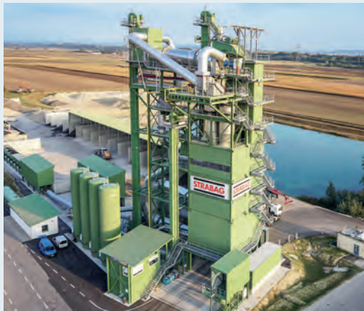
The asphalt mixing plant processes up to 50 % recycling material.
