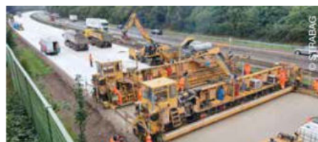
Widening of the A1 motorway.
