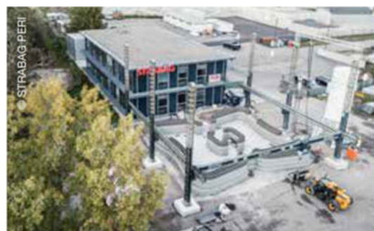
Pioneer in concrete printing.
