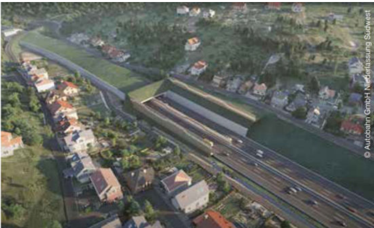
Large-scale project Enz Valley crossing
