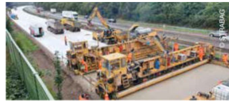
Widening of the A1 motorway.
