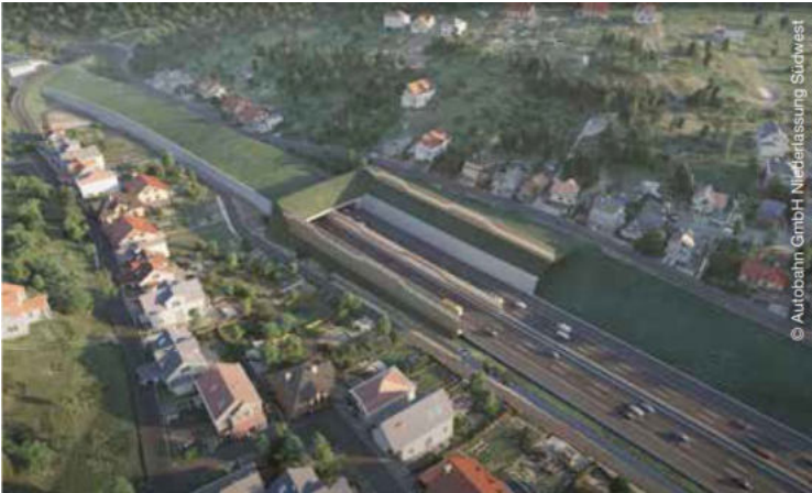
Large-scale project Enz Valley crossing
