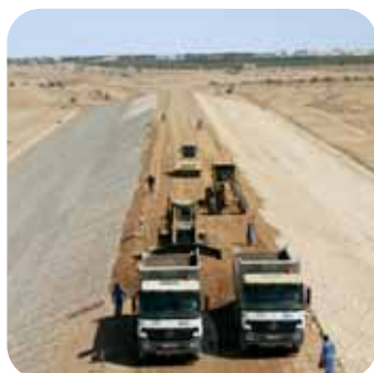
Left: Finishing the dam crest
