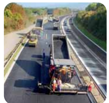
Site manageress Stefanie Führling explains the construction schedule Paving – hot on hot – on federal motorway A 602 Trier in staggered shifts
