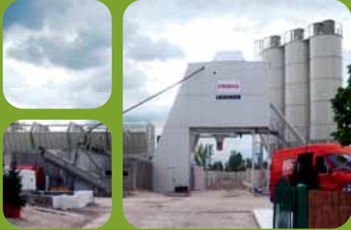
Supplying a mixing plant
