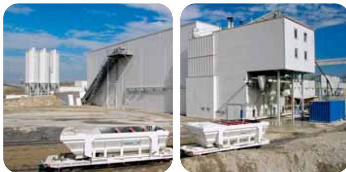
Mixing plant at the Wienerwaldtunnel West site
