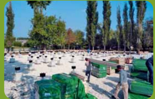
A social center construction site
