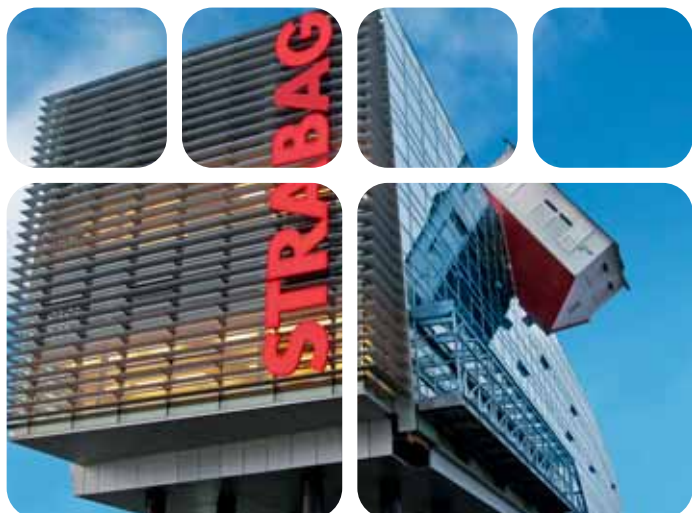
STRABAG head office in Bratislava under attack
