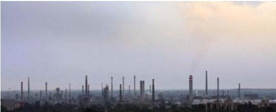
Slovakia, SlovNaft, (Petrochemical refinery), Bratislava
