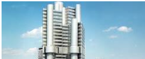
HVB Tower, Munich
