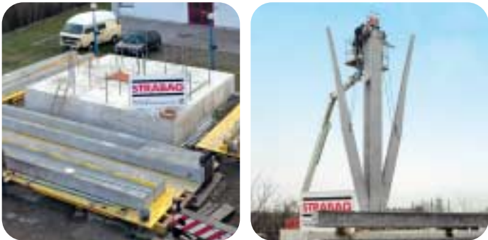
3 parts of the bridge before final assembly.
