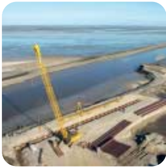
Sheet-pile walls at the port entrance.
