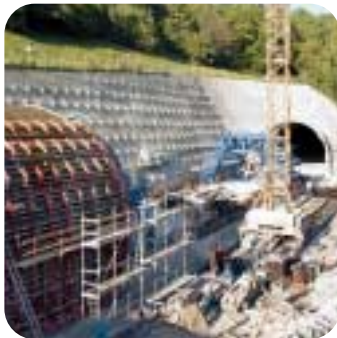
Left: The tunnel from outside.
