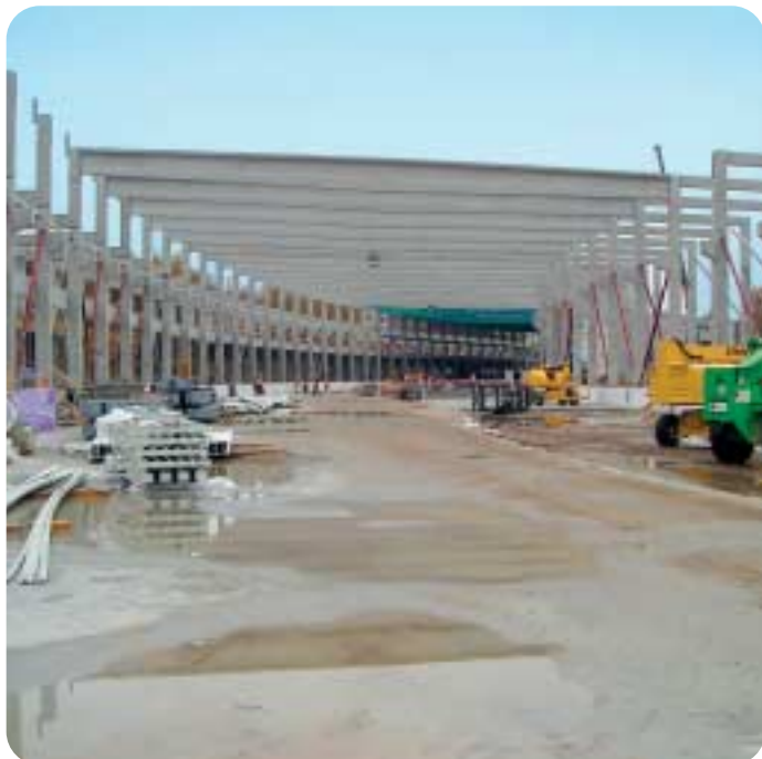
The research center's walls and ceiling are being mounted.
