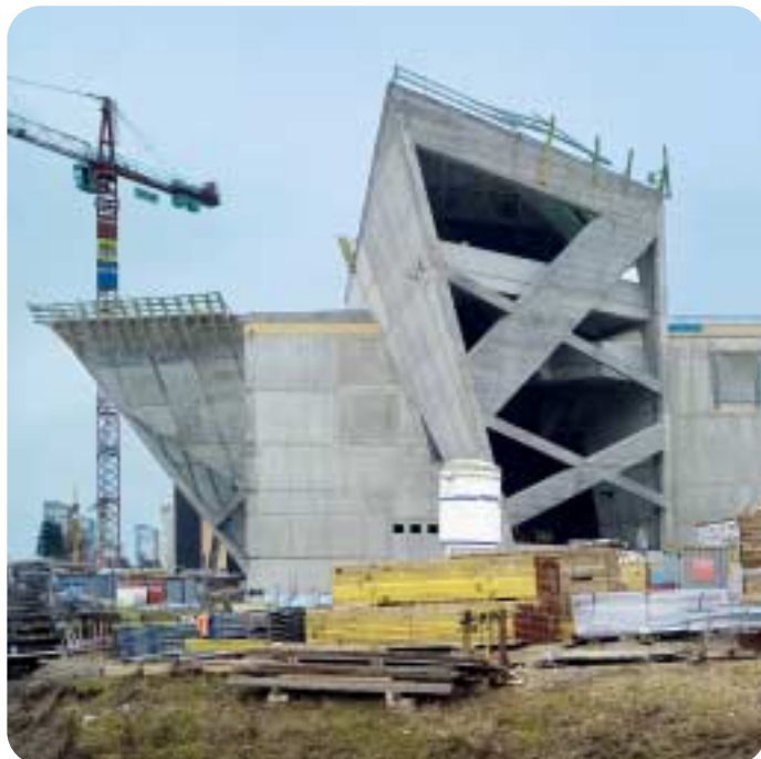
85,000 m 3 of enclosed space are being created.
