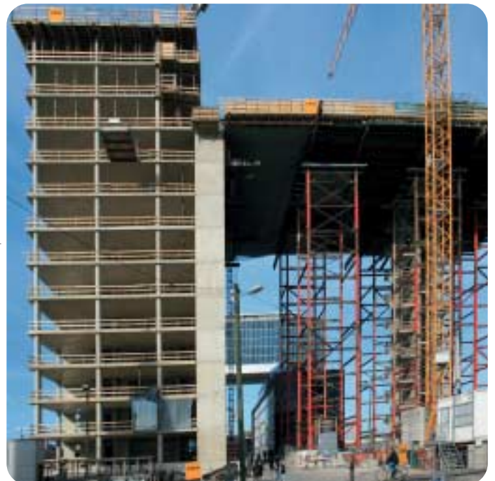
All in all, 17 storeys and a basement are to be erected.
