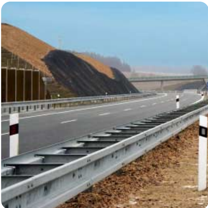
Seven bridges and three flyovers had to be built, as well.
