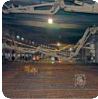
Left: Several pumps were used for pouring the concrete. Right: A close-up of the concreting works.
