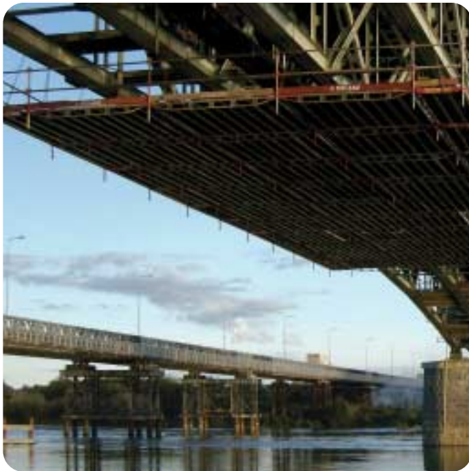
The new bridge is taking shape.
