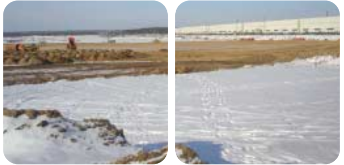
Here, the Vyksa steel plant will soon be taking shape.
